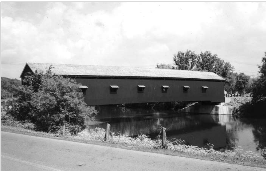
Buskirks Bridge, rebuilt 2004. First bridge here built in 1804, serving the Great Northern Turnpike, by Martin Buskirk, a tavern-keeper on the Cambridge, New York, side of the Hoosick River, re-built about 1850.
